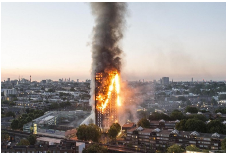
A blaze rages through Grenfell Tower block in Notting Hill, London 2017. Photo: Jeremy Selwyn, source: facebook
